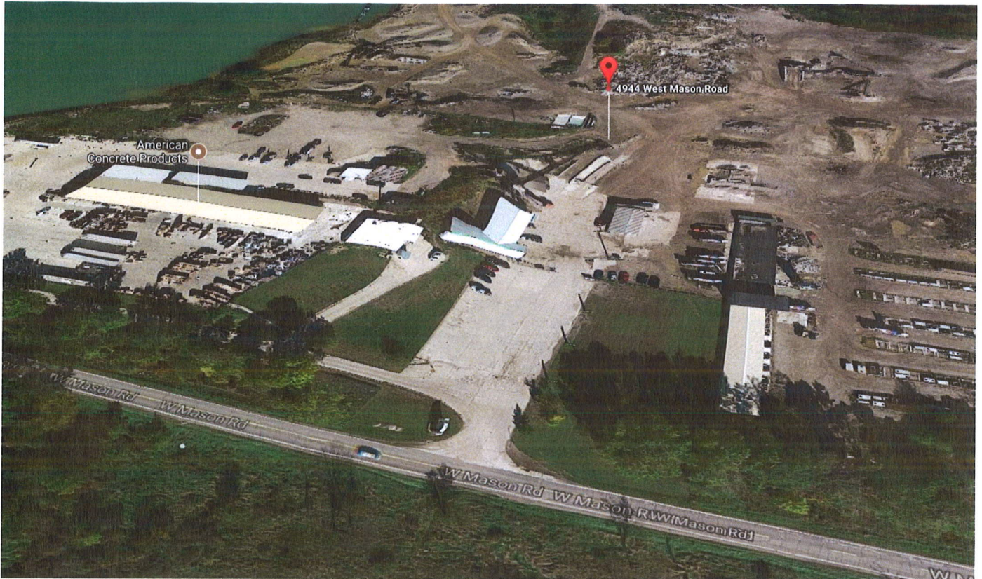
Aerial view from Mason Road
