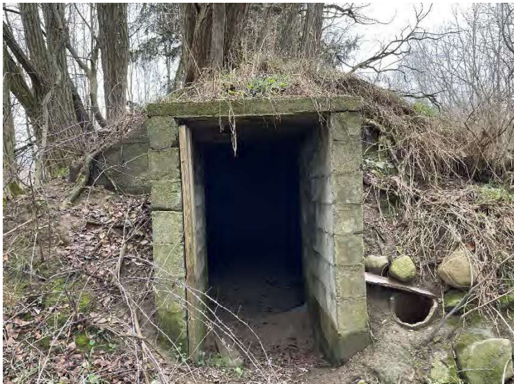
Photo 17. Shelter with vent
