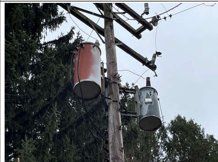
Photo 5. Pole-mounted transformers
