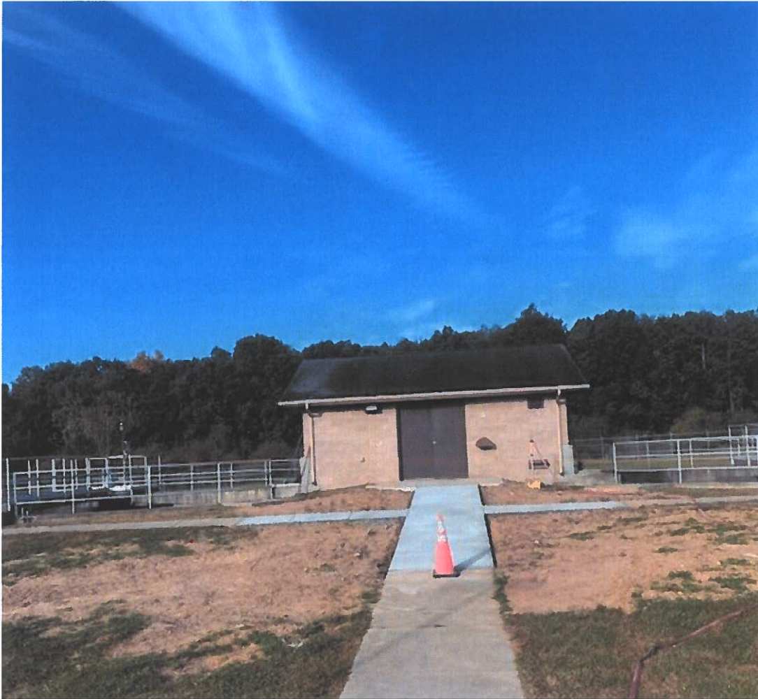
Concrete Sidewalk Restoration
