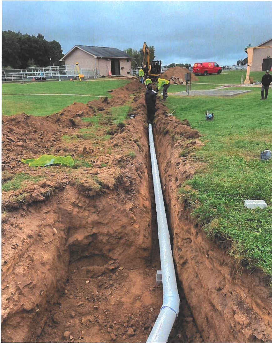
Clarifier Drain Line Installation
