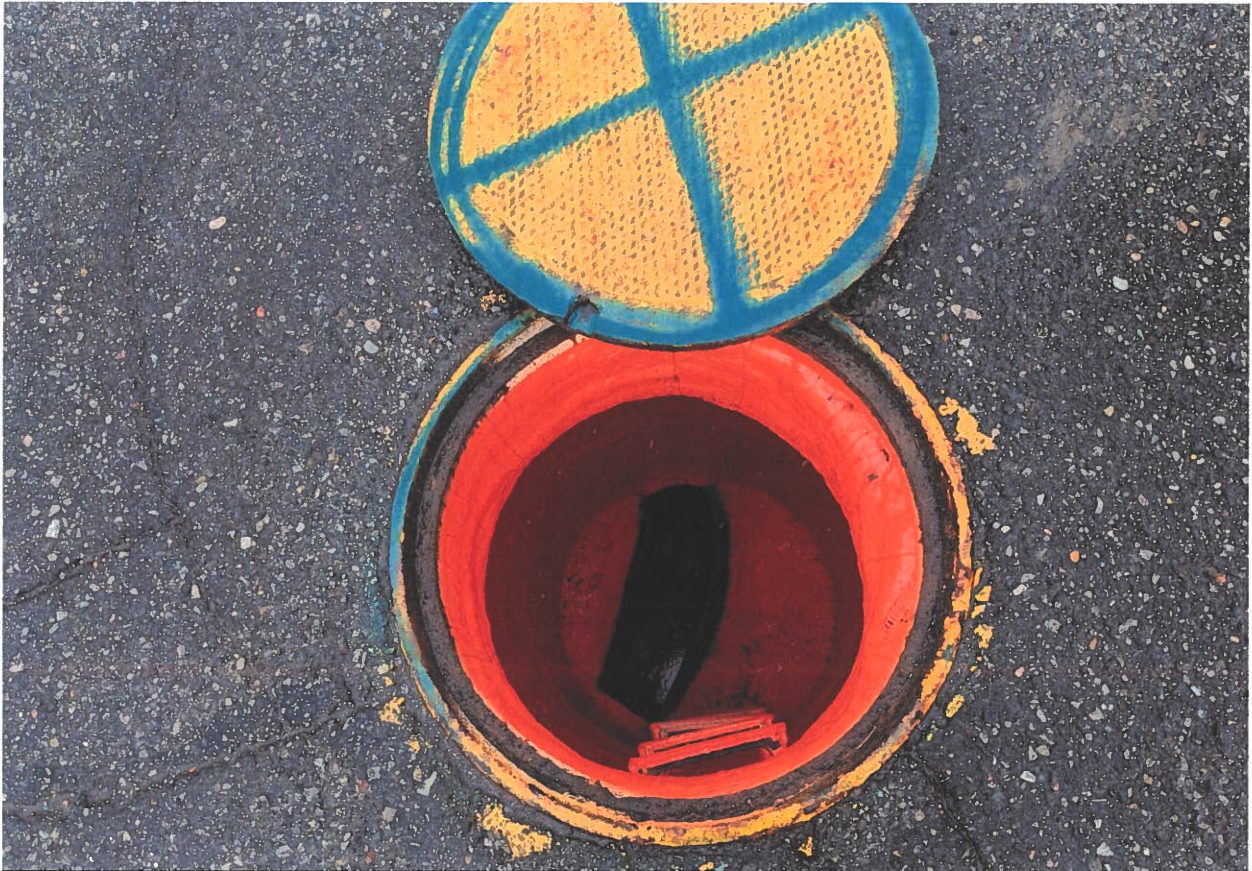
Manhole HSMH-0062 After Lining
