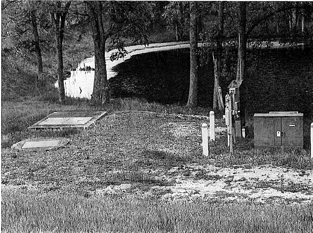
Pump Station 77 at Operating Engineer's Facility
