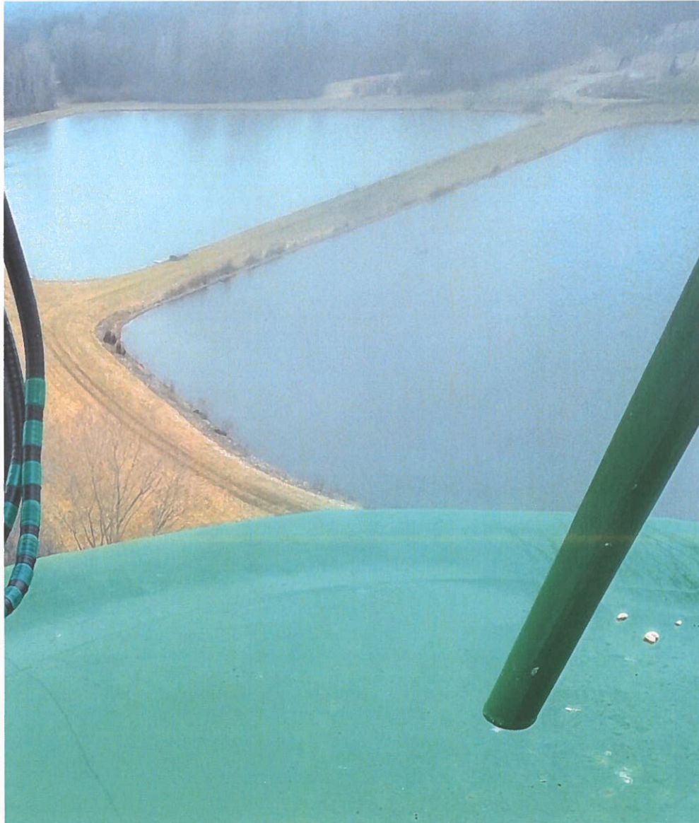
Howell Township WWTP from Trans West Tower
