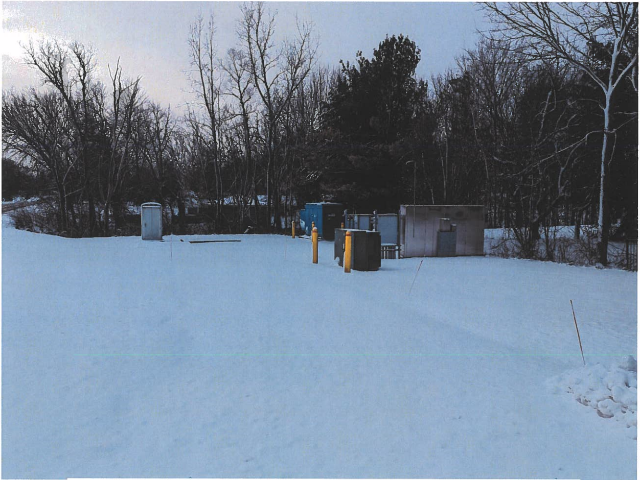
Pump Station 75 – Oak Grove Road
