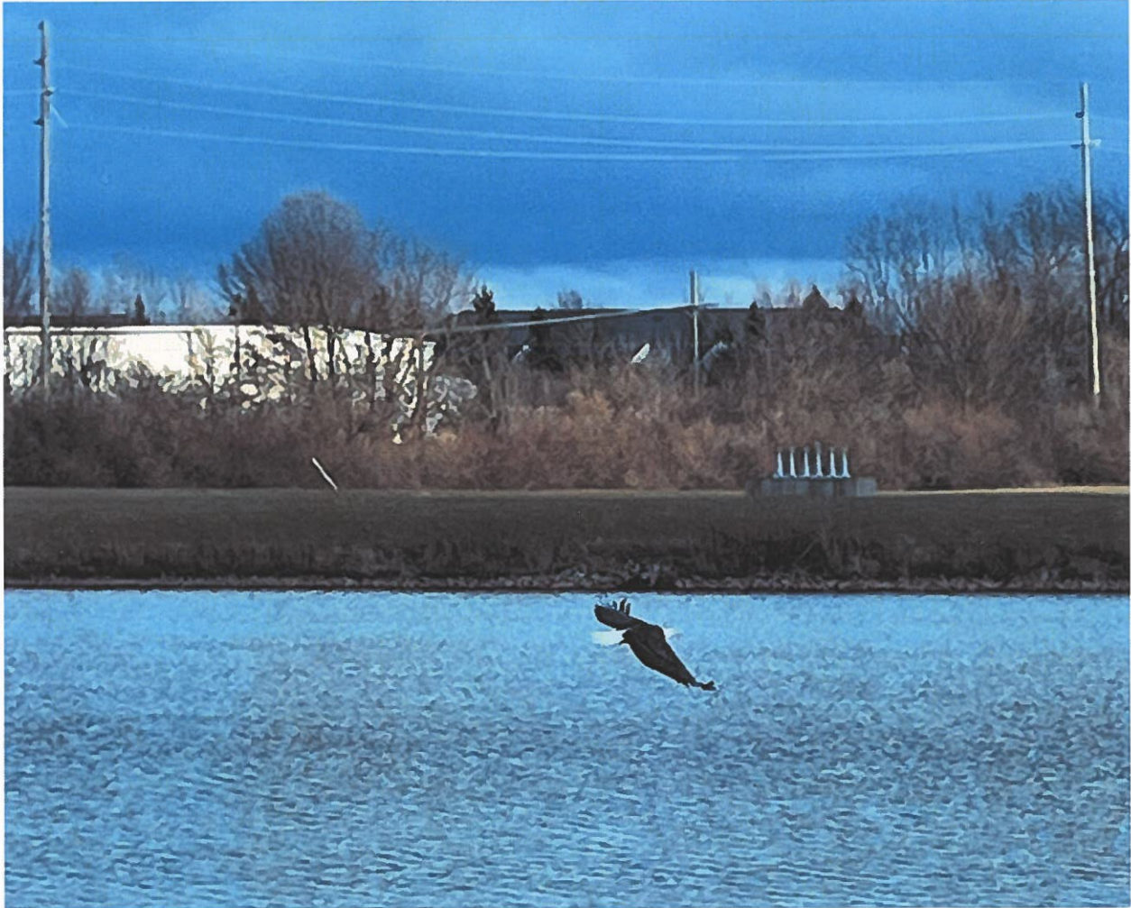
Eagle Flying Over Lagoons at WWTP
