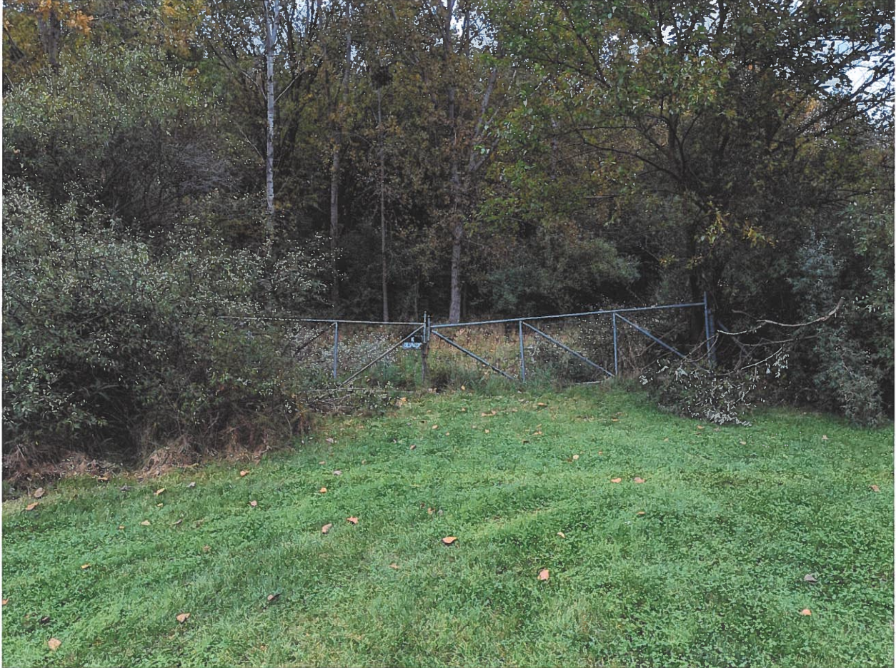
Gate On East Side of Property – Discharge Effluent Pipe Easement
