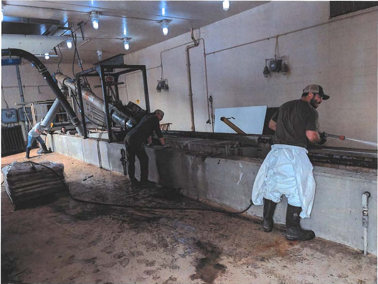
Cleaning of Headworks Building Prior to Lining
