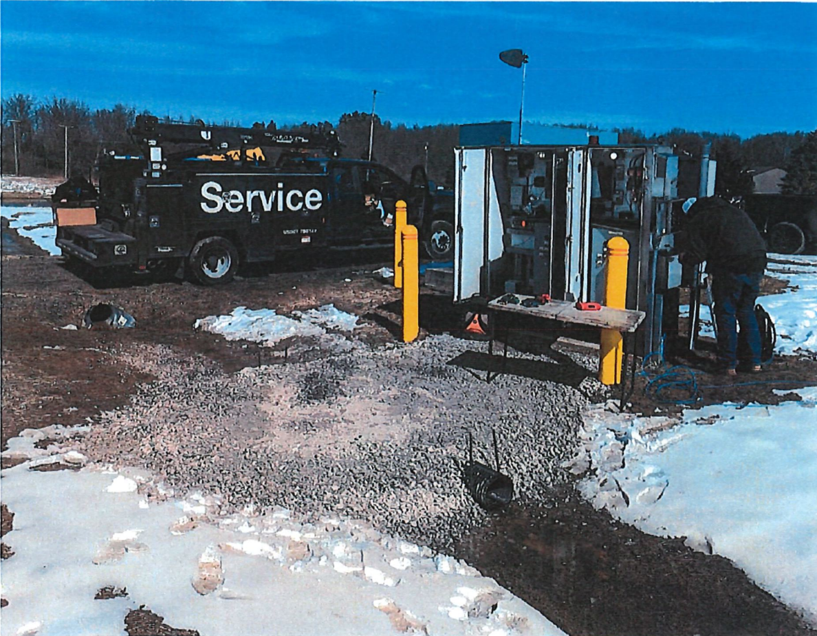
Station 76- Kennedy Installing KISM and Gravel and Culvert
