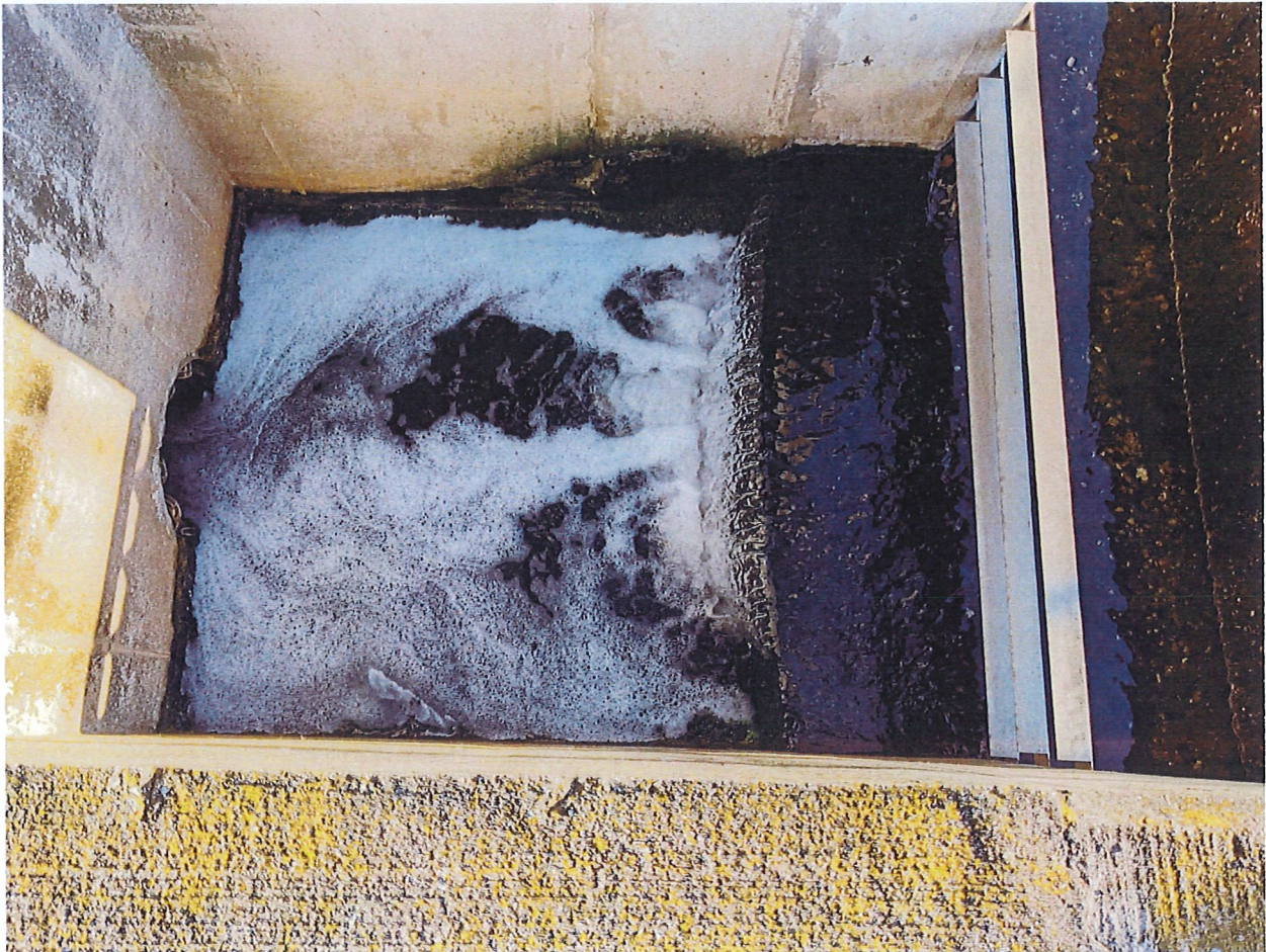
Howell Township Secondary Clarifier Effluent – November 9, 2022
