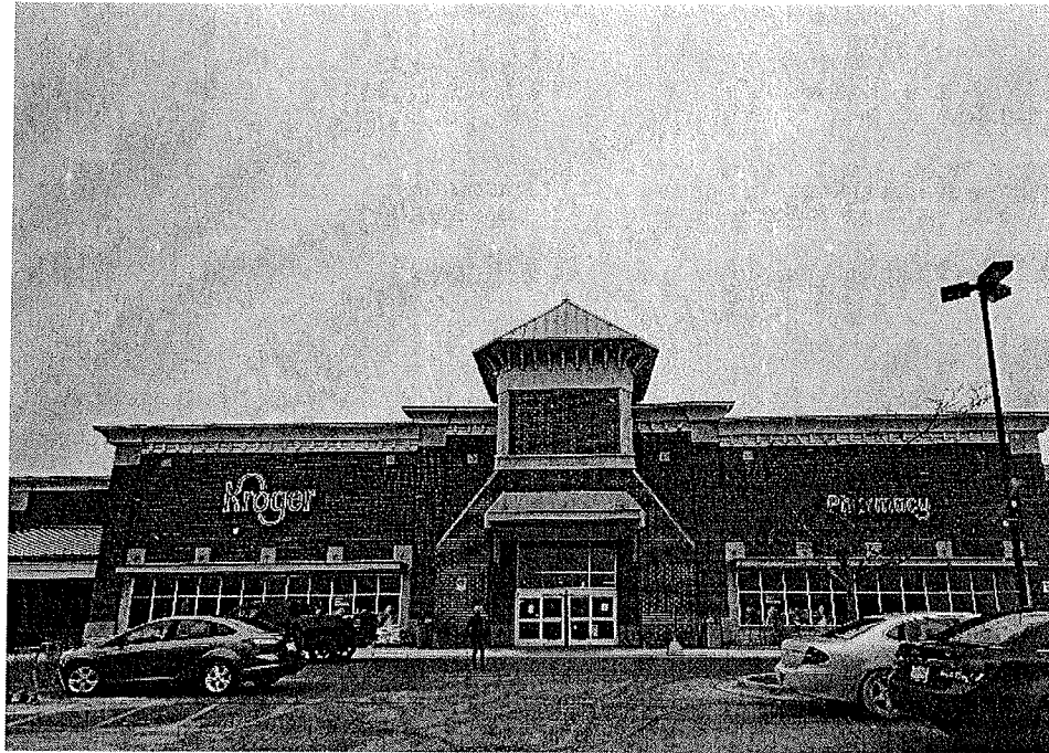
Kroger, South of Subject Lot, in Strip Mall Shopping Center off West Highland Road
