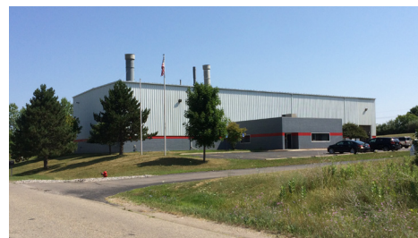
Typical Industrial Facility
