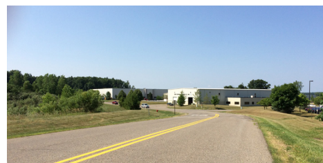
Typical Business Park
