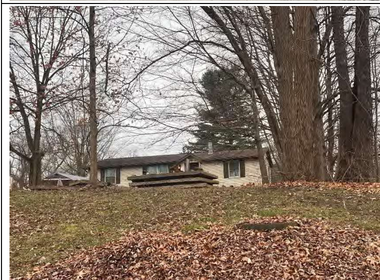
Photo 24. South adjoining, residence
