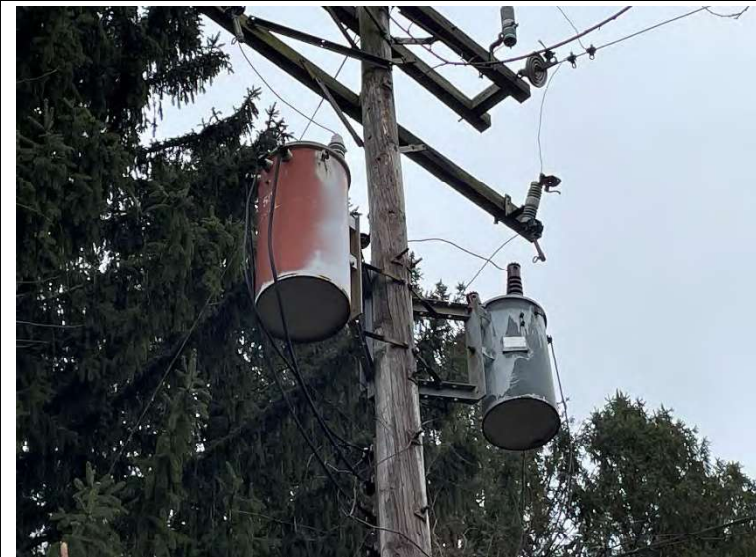
Photo 5. Pole-mounted transformers
