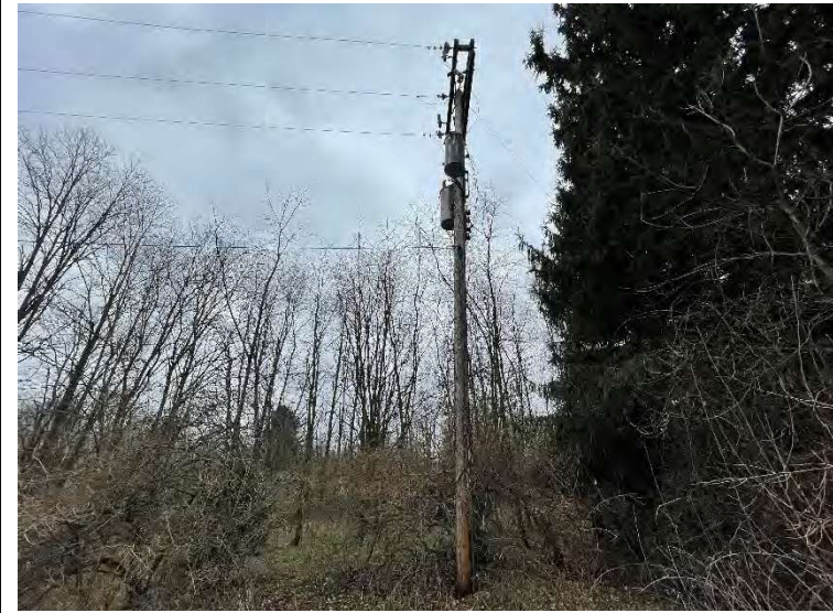
Photo 4. Pole-mounted transformers
