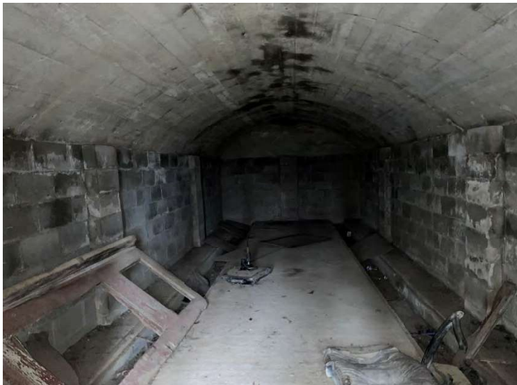
Photo 18. Inside of shelter
